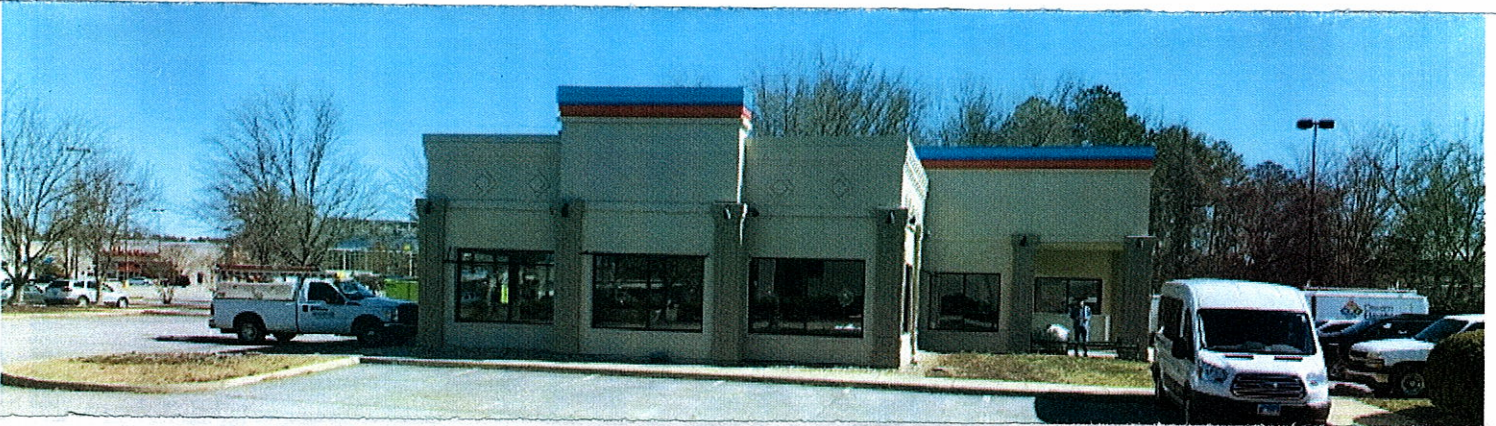
1101 Carmia Way used to be home to a Ruby Tuesday. It's being transformed into an IHOP, which is set to open in April. (Photo: D'Andre Henderson)
